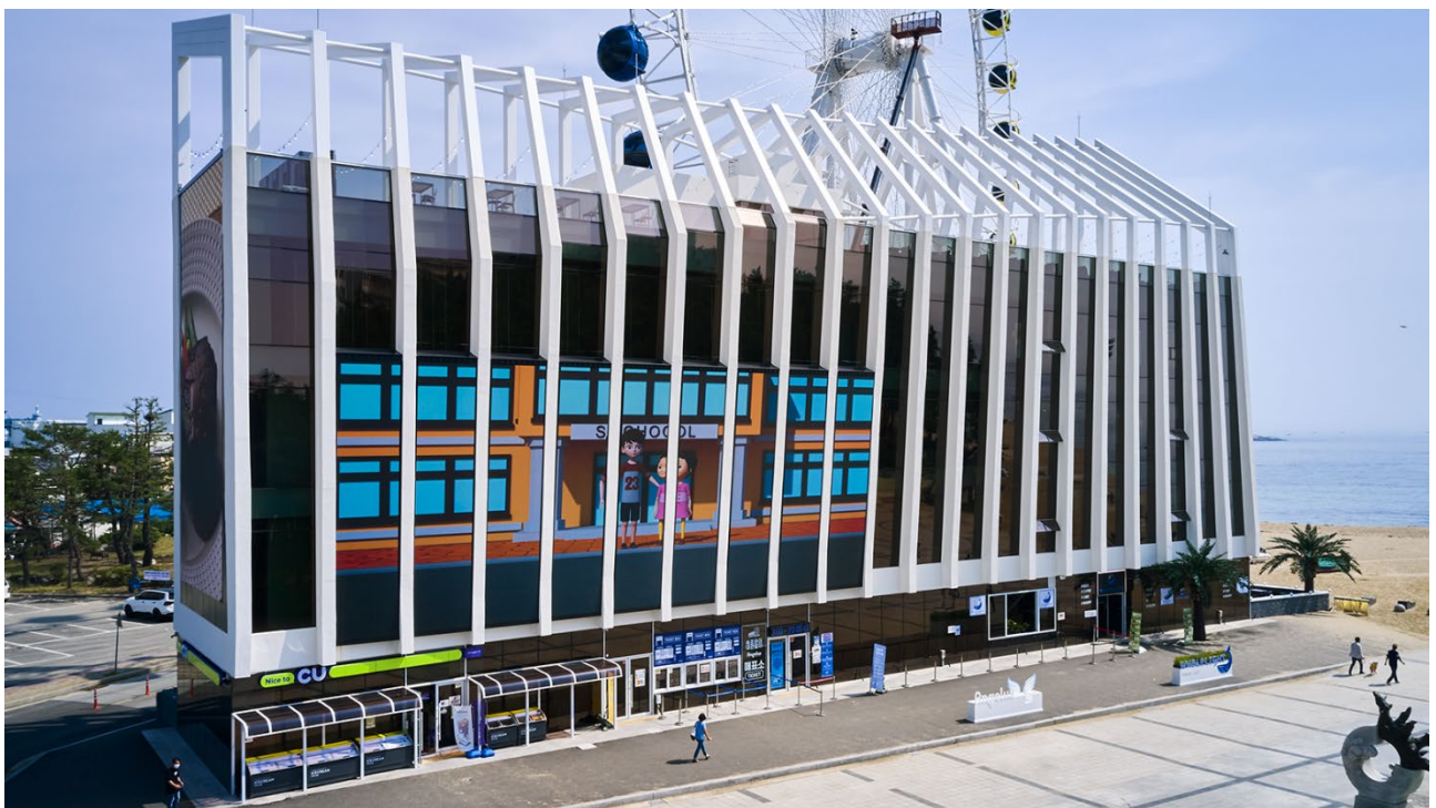
Aluminum screen on the south side of Sokcho coast, Gangwon-do, South Korea (150m 2 )
